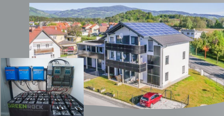
24 kWh system in a house with 8 apartments in Styria, Austria
